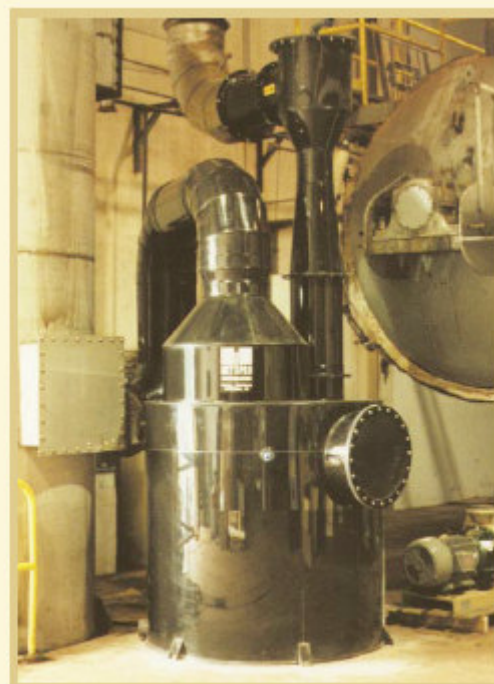
Fig 18: Venturi gas scrubber
